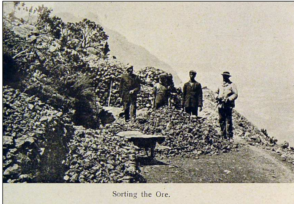
Figure 7 : Sorted and stacked manganese ore probably located below the open workings (see Fig. 2). Sourced from the Cape Argus Weekly, dated 26 th January 1910.
