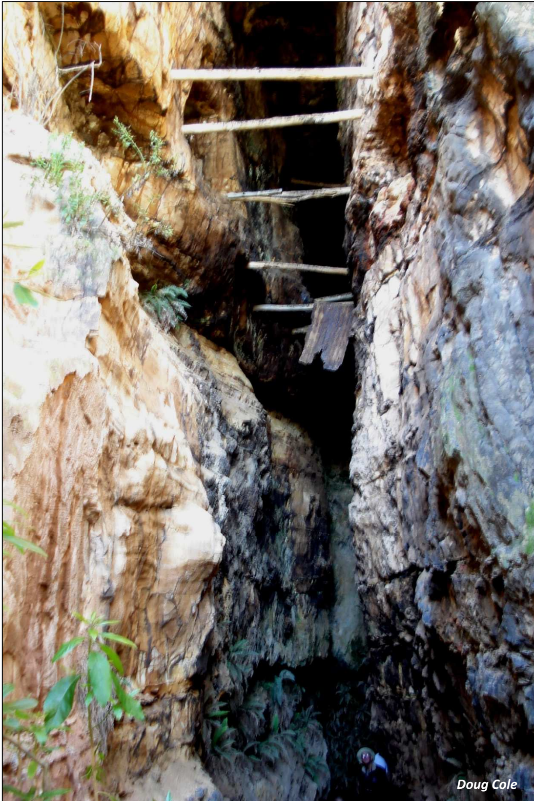
Figure 11 : Lowermost adit showing horizontal timber supports and rusted corrugated iron. A picture of the actual mining in this adit in January 1910 is shown in Fig. 4. (for location see Fig. 2).
