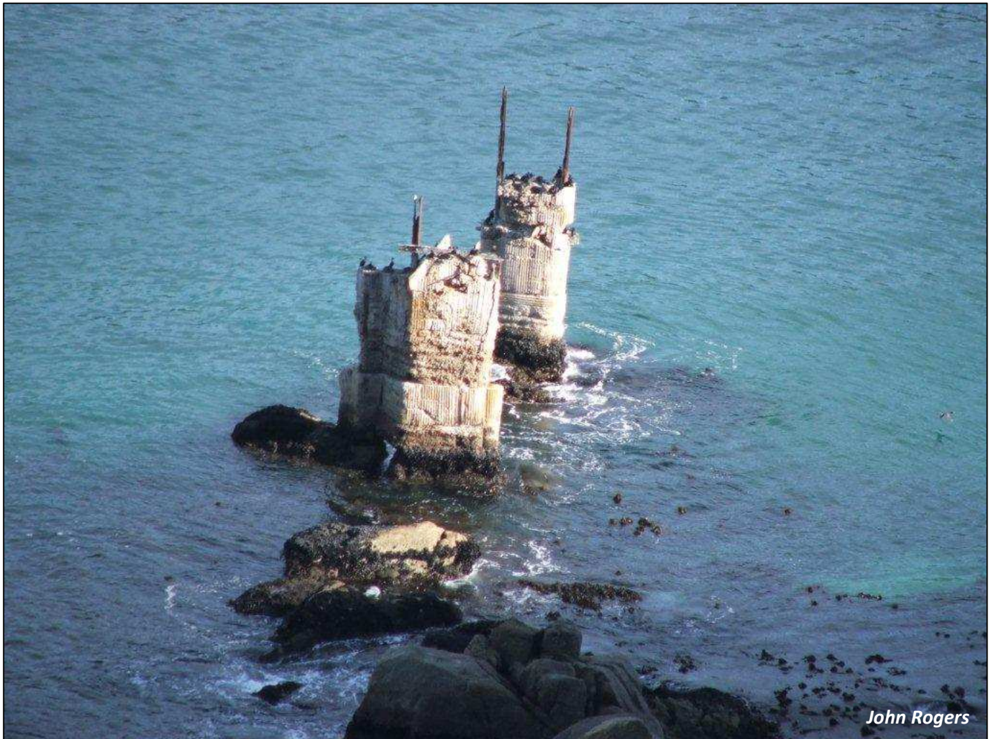
Figure 13 : Two concrete pillars, standing in the sea below the Chapman's Peak Drive, about 350 m northwest of East Fort (see Fig. 2). These pillars represent the only remaining part of the jetty that was used for the shipment of manganese ore (see Fig. 10).
