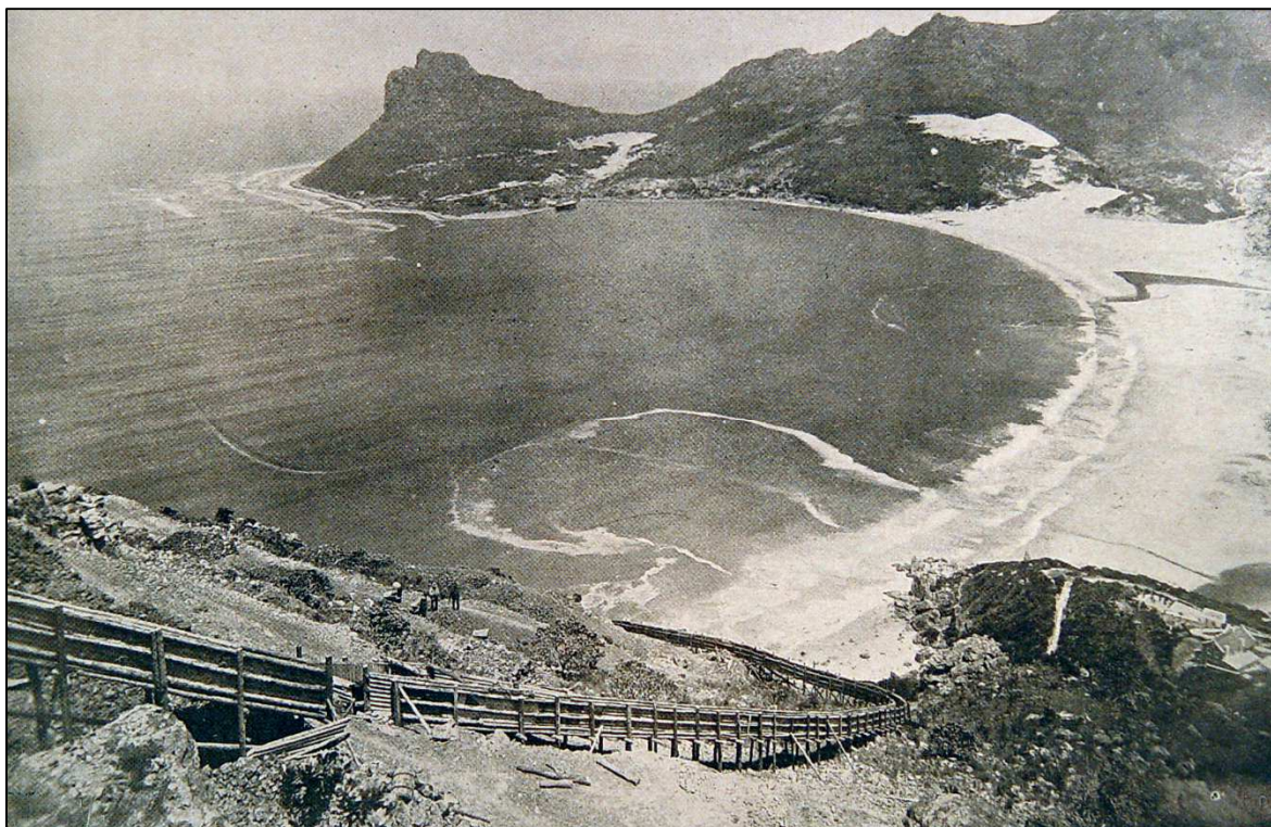
Figure 8 : Manganese chute high up on slopes above Hout Bay with a loading station in the foreground that probably received ore from the adits (see Figs. 3 and 5). Note the plume of disturbed water resulting from a large rip current off Flora Bay. Sourced from the Cape Argus Weekly, dated 26 th January 1910.
